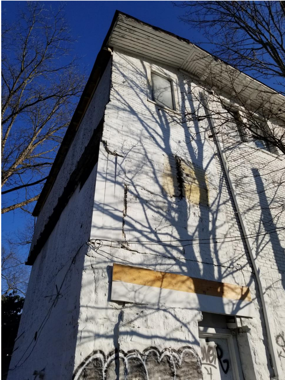
#16 – Rear portion of left side (west – Argonne Ave, NE) façade, looking southeast
