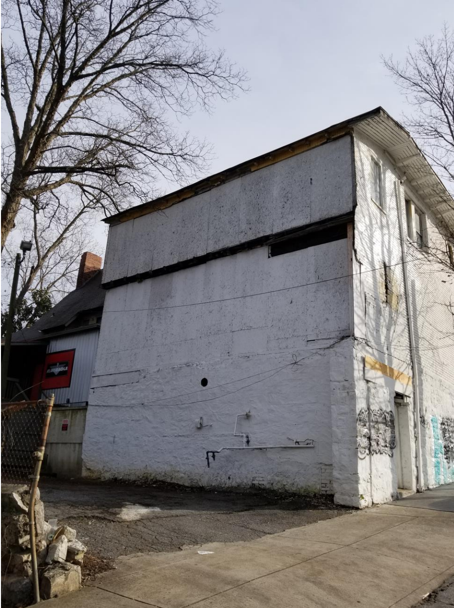
#19 – Rear (north) façade, looking southeast
