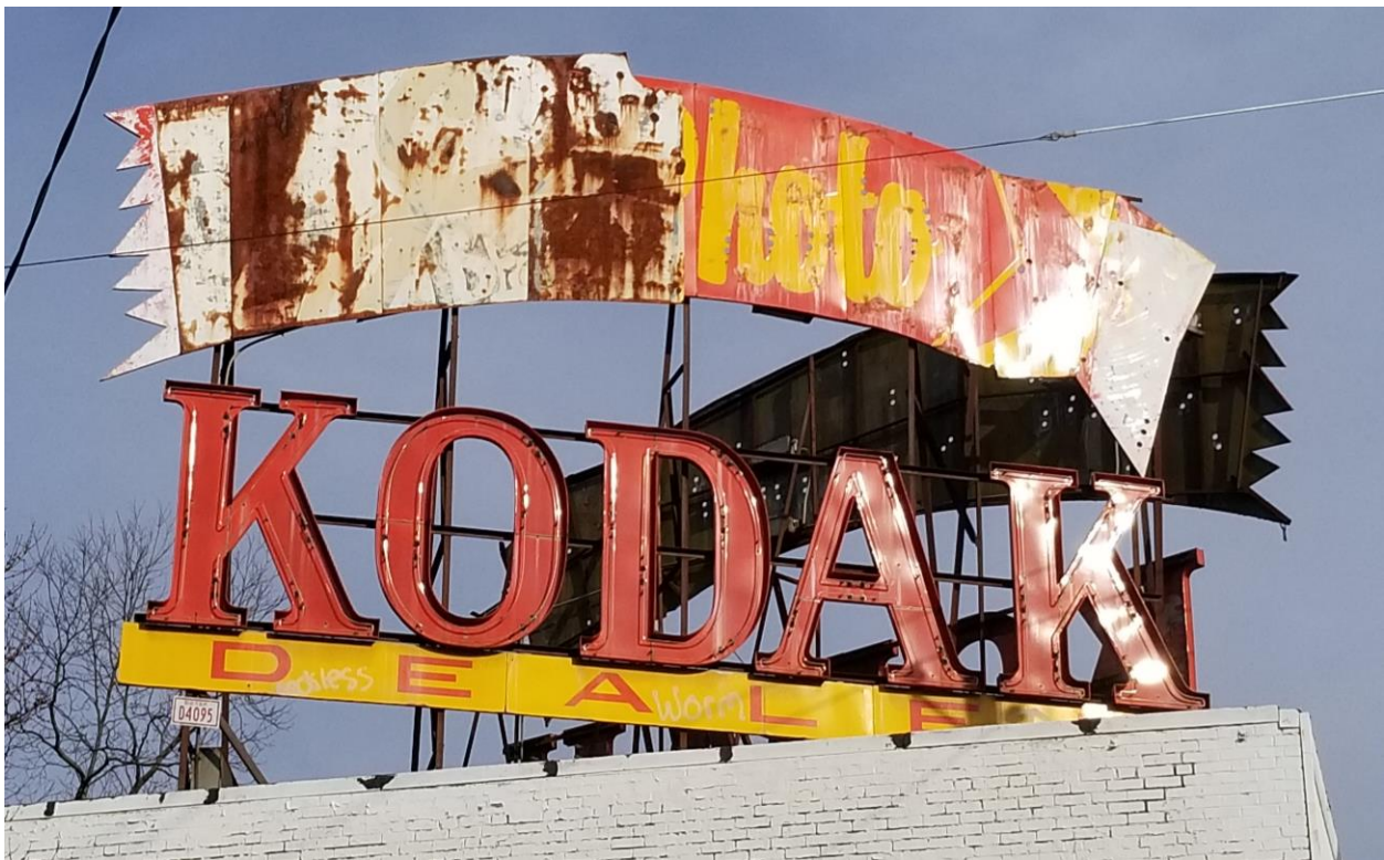
#9 – Rooftop signage, western face, looking northeast
