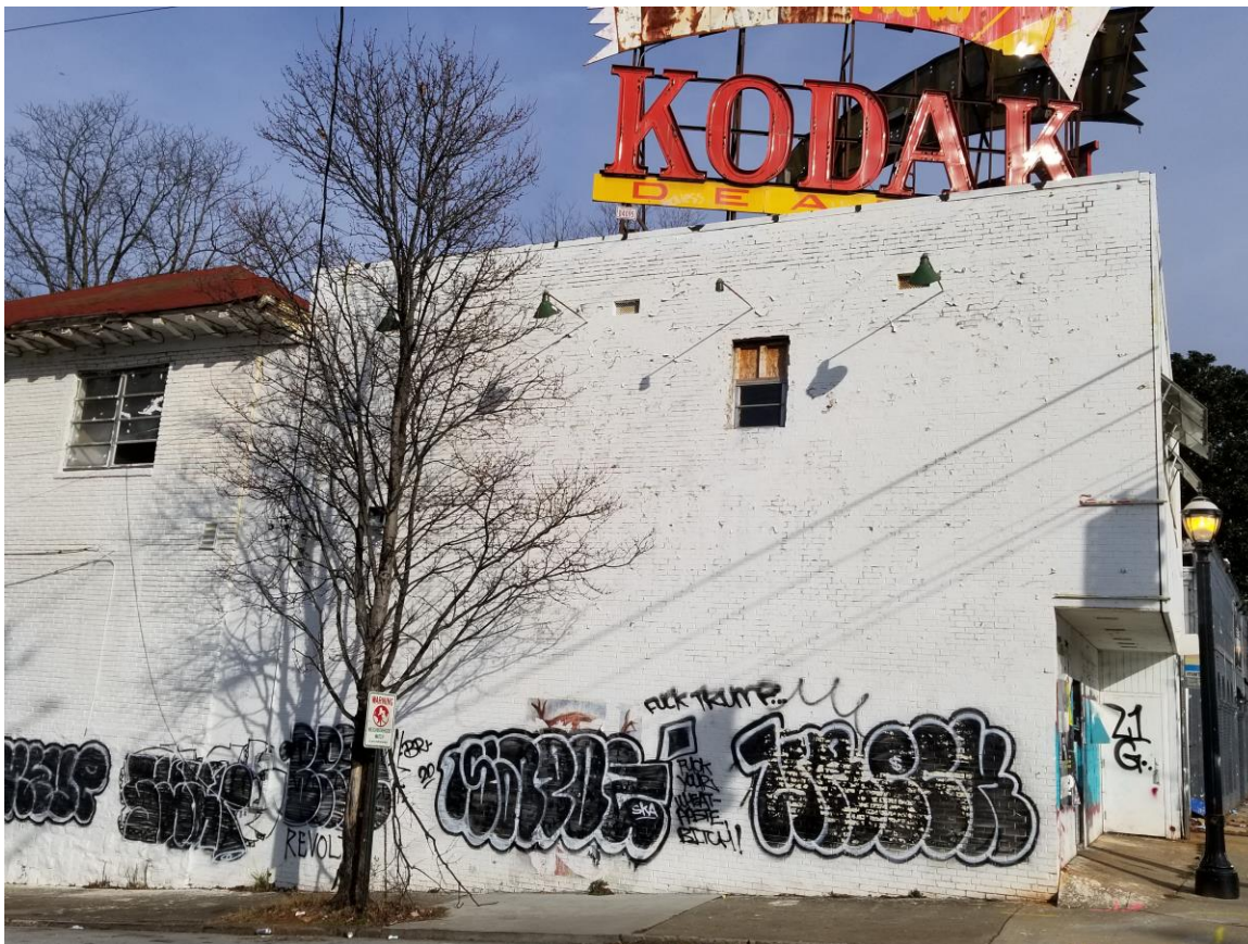
#11 – Front portion of left side (west – Argonne Ave, NE) façade, looking east
