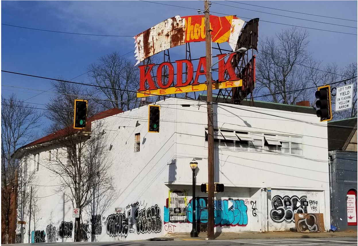
#1 – Front (south – Ponce de Leon Ave, NE) and left side (west – Argonne Ave, NE) facades, looking northeast
