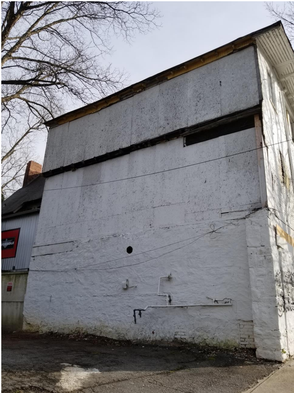
#18 – Rear (north) façade, looking southeast
