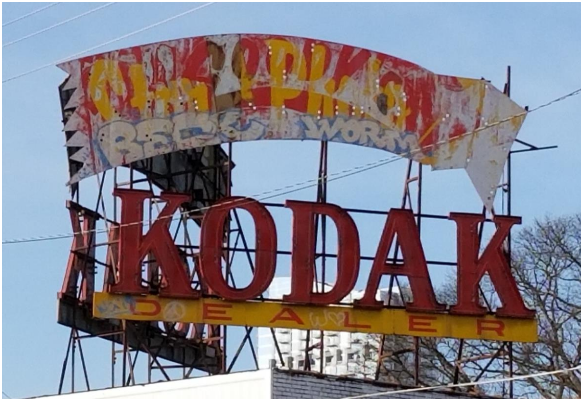
#10 – Rooftop signage, eastern face, looking northwest
