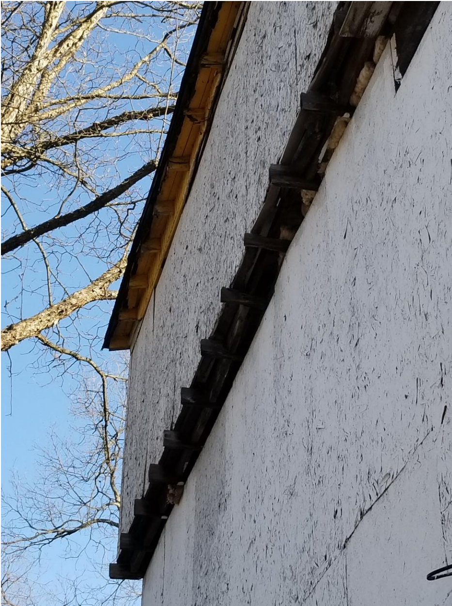
#21 – Rear (north) façade and eave detail, looking east
