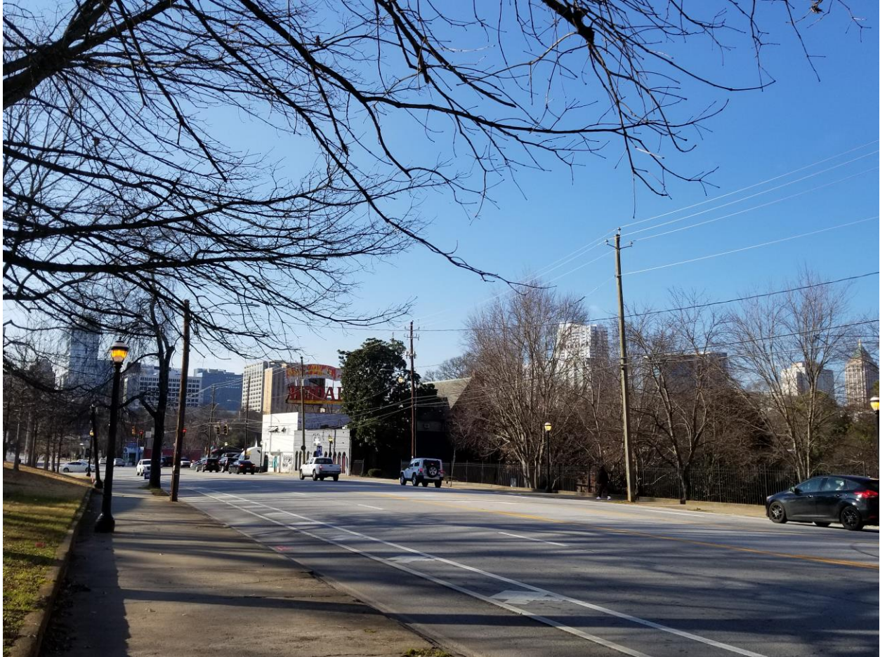
#25 – Front (south – Ponce de Leon Ave, NE) façade and adjacent Atlanta Eagle Building, looking northwest from Ponce de Leon Avenue, NE
