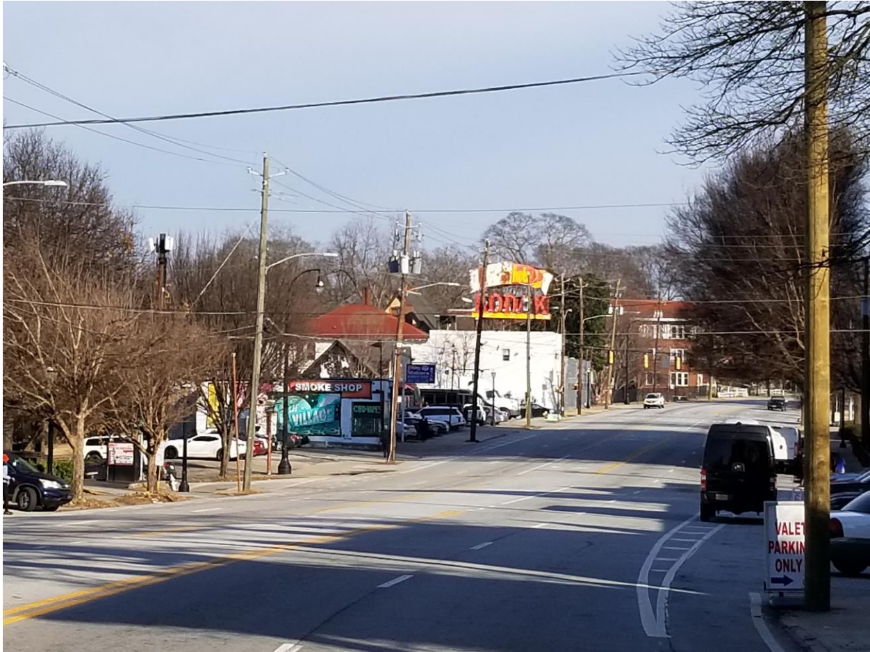
#27 – Left side (west – Argonne Ave, NE) and front (south – Ponce de Leon Ave, NE) facades, looking northeast from Ponce de Leon Ave, NE
