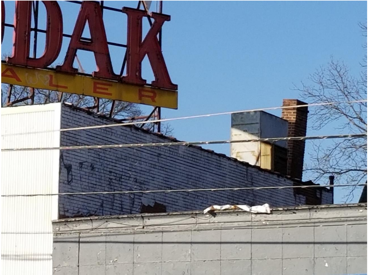
#22 – Right side (east) façade, looking northwest
