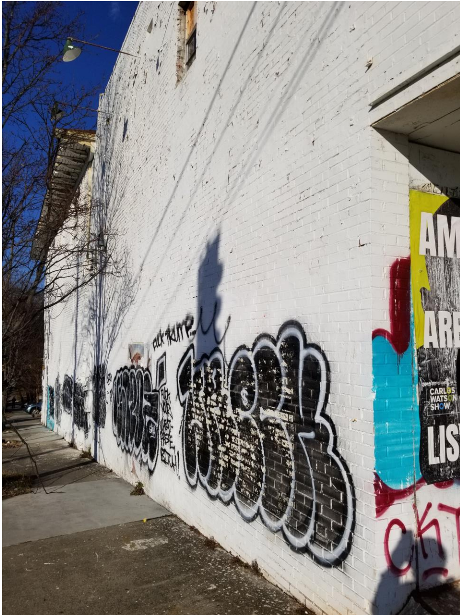
#13 – Left side (west - Argonne Ave, NE) façade, looking northeast
