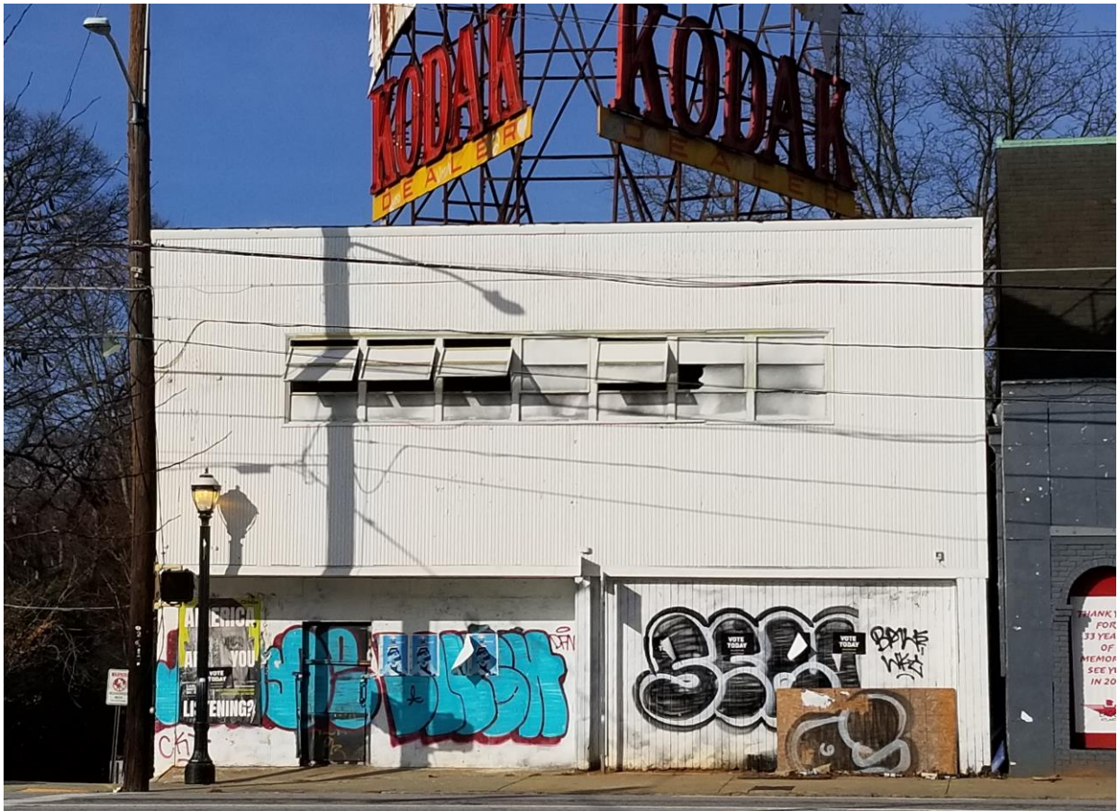
#2 – Front (south – Ponce de Leon Ave, NE) façade, looking north
