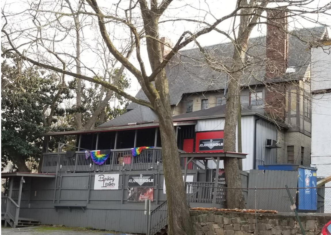
#16 – Rear (north) and left side (west) facades, looking southeast
