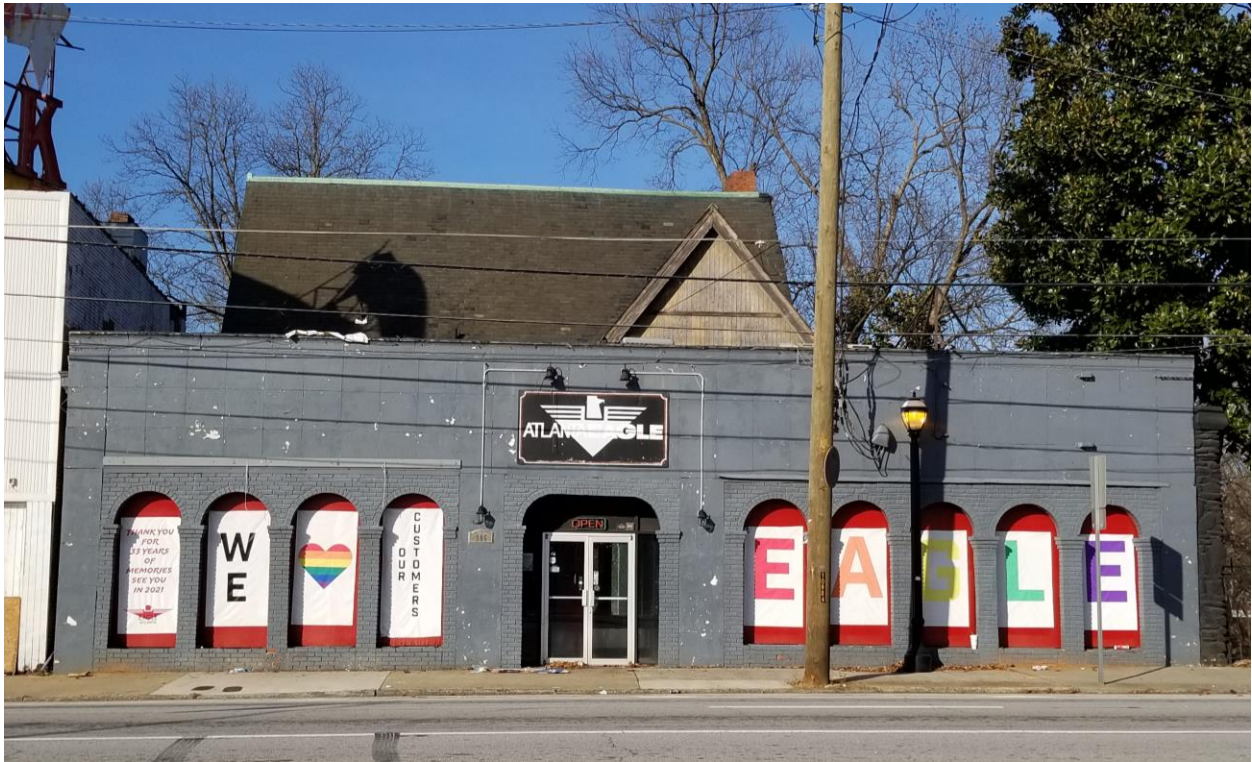
#1 – Front (south – Ponce de Leon Ave, NE) façade, looking north
