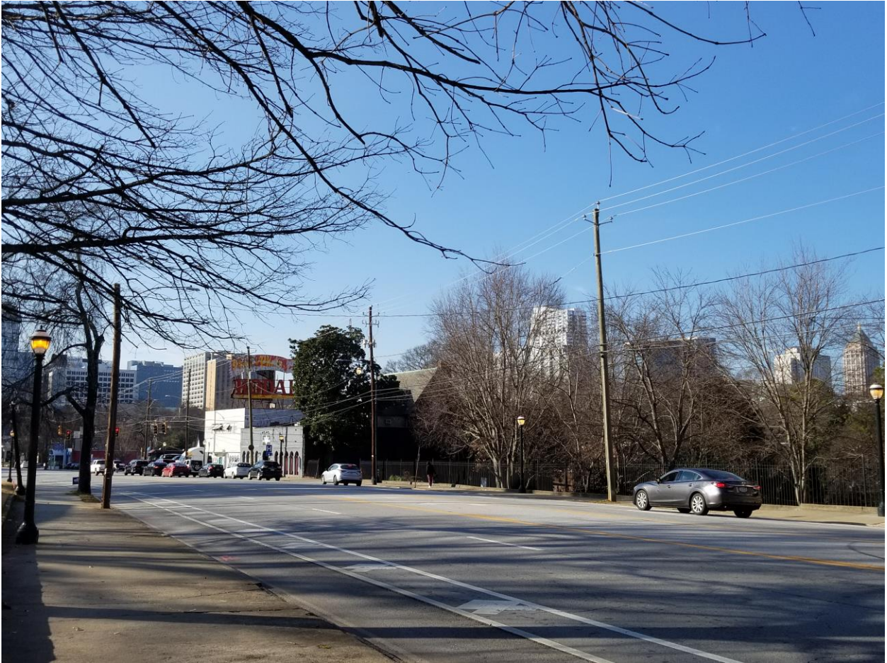
#29 – Front (south – Ponce de Leon Ave, NE) and right side (east) façades and adjacent Kodak Building, looking northwest from Ponce de Leon Avenue, NE
