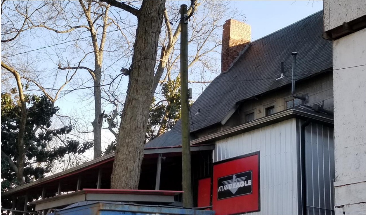
#20 – Upper portion of rear (north) facade, looking southeast
