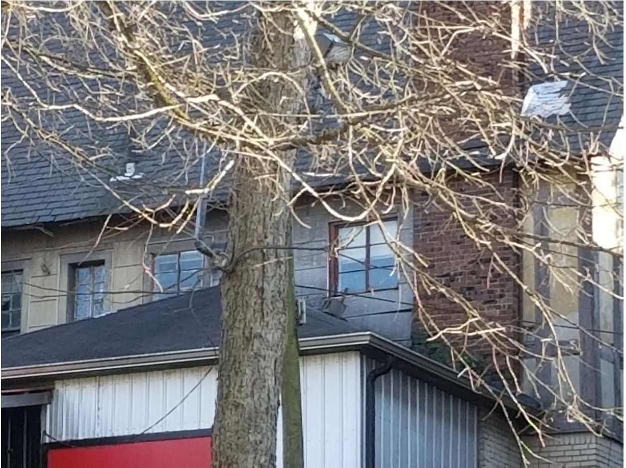
#22 – Upper portion of rear (north) facade, looking southeast
