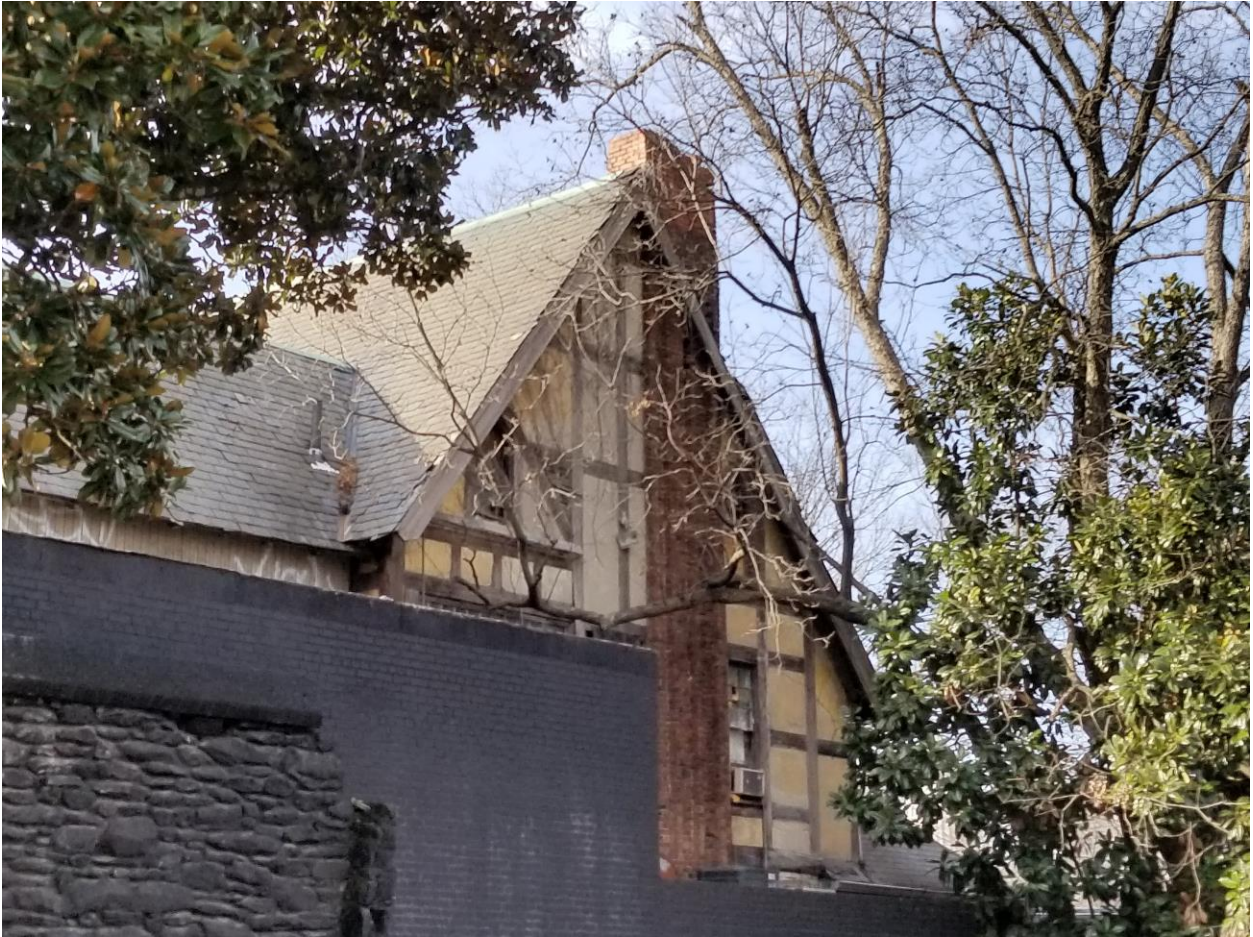
#13 – Rear portion of right side (east) façade, looking northwest
