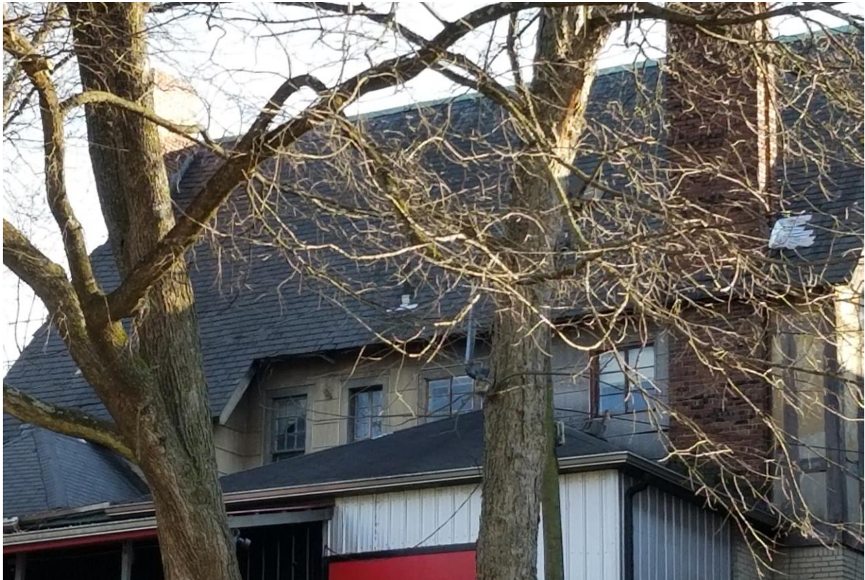
#21 – Upper portion of rear (north) facade, looking southeast
