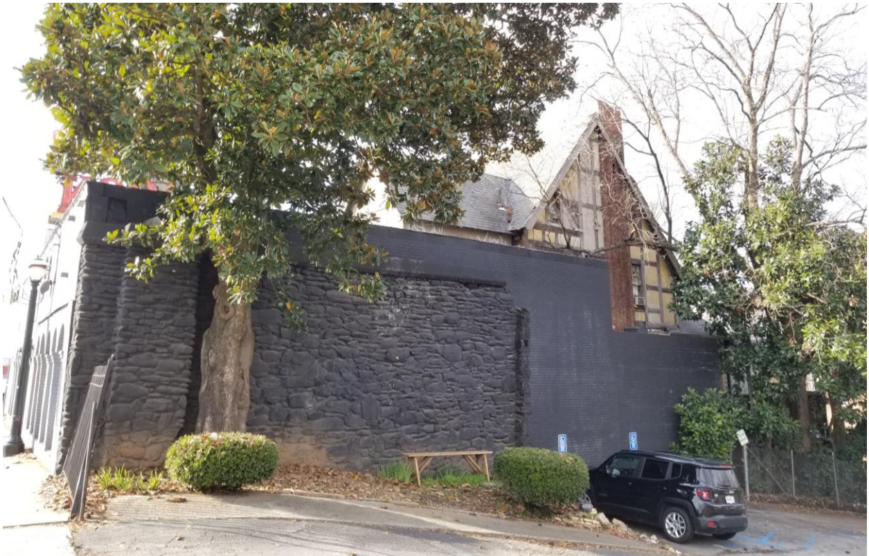
#12 – Right side (east) façade, looking northwest
