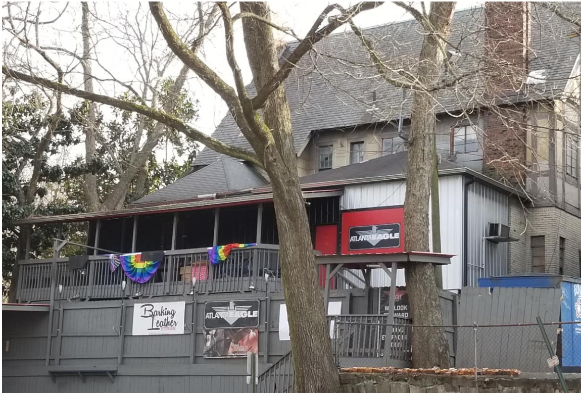
#17 – Rear (north) and left side (west) facades, looking southeast
