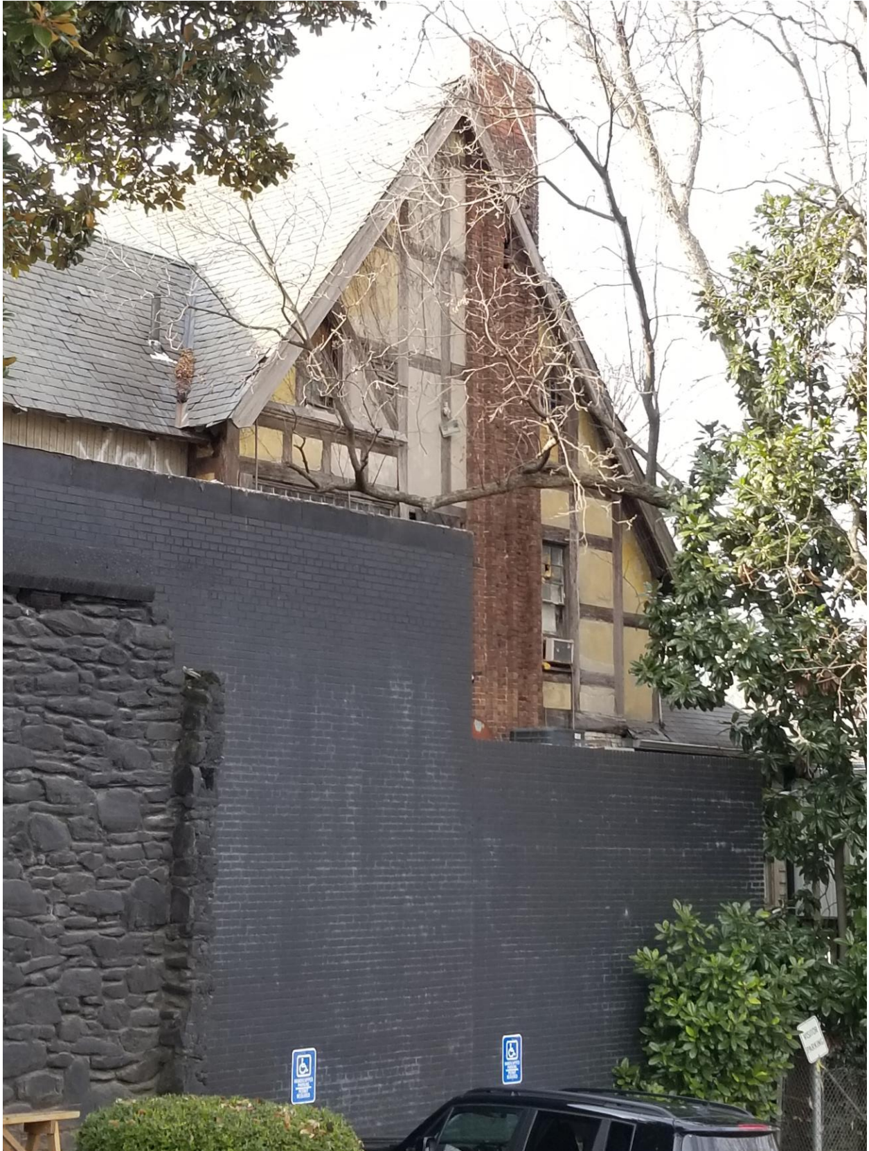
#14 – Rear portion of right side (east) façade, looking northwest
