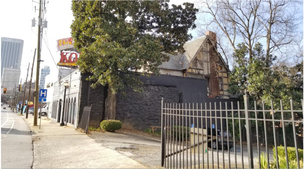
#11 – Right side (east) façade, looking northwest
