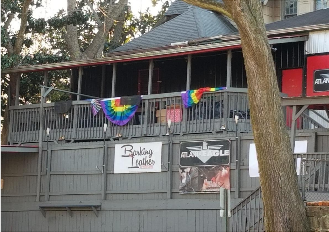
#18 – Rear (north) and left side (west) facades, looking southeast
