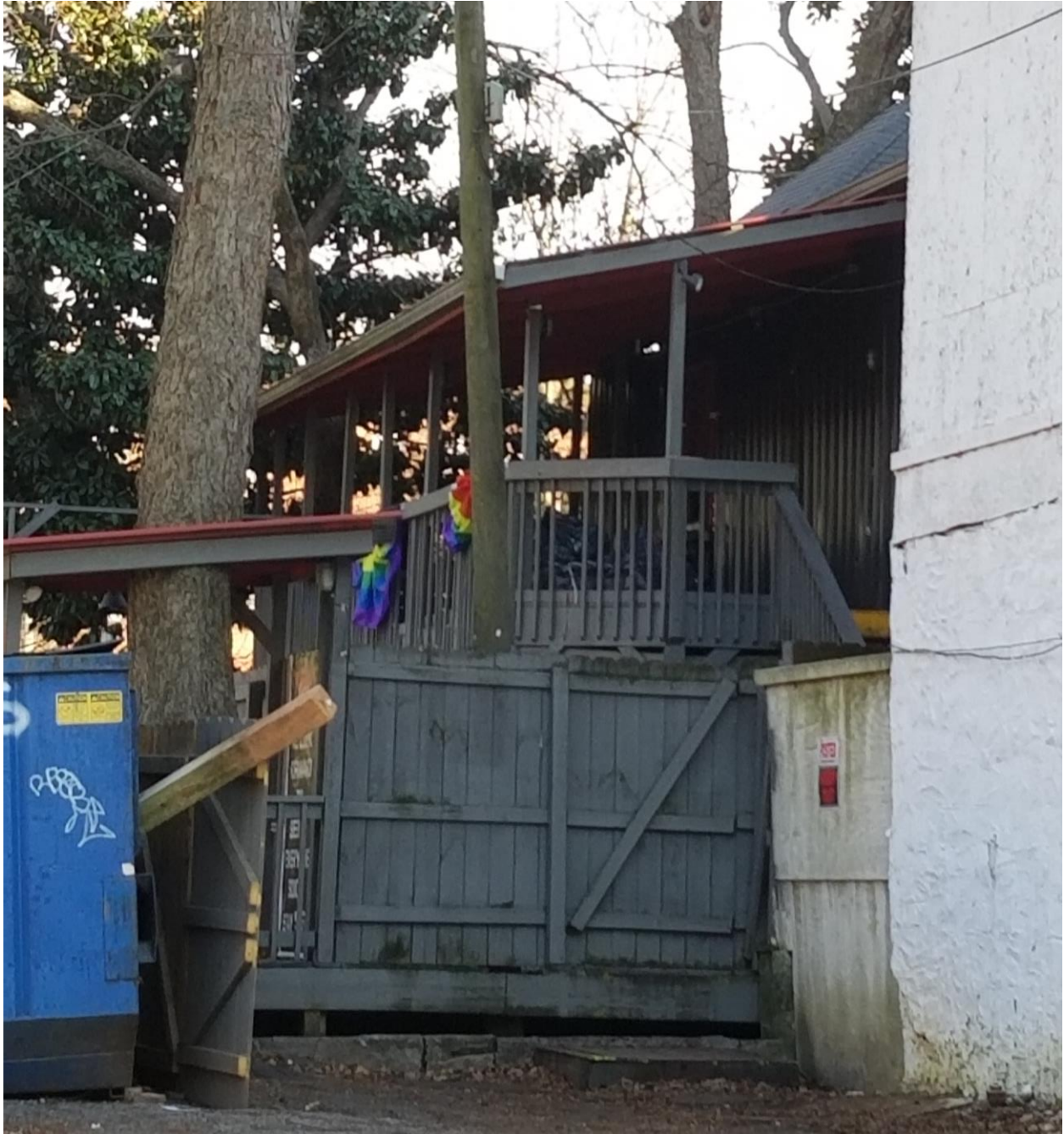
#24 – Rear (north) façade, looking east with Kodak Building property in foreground
