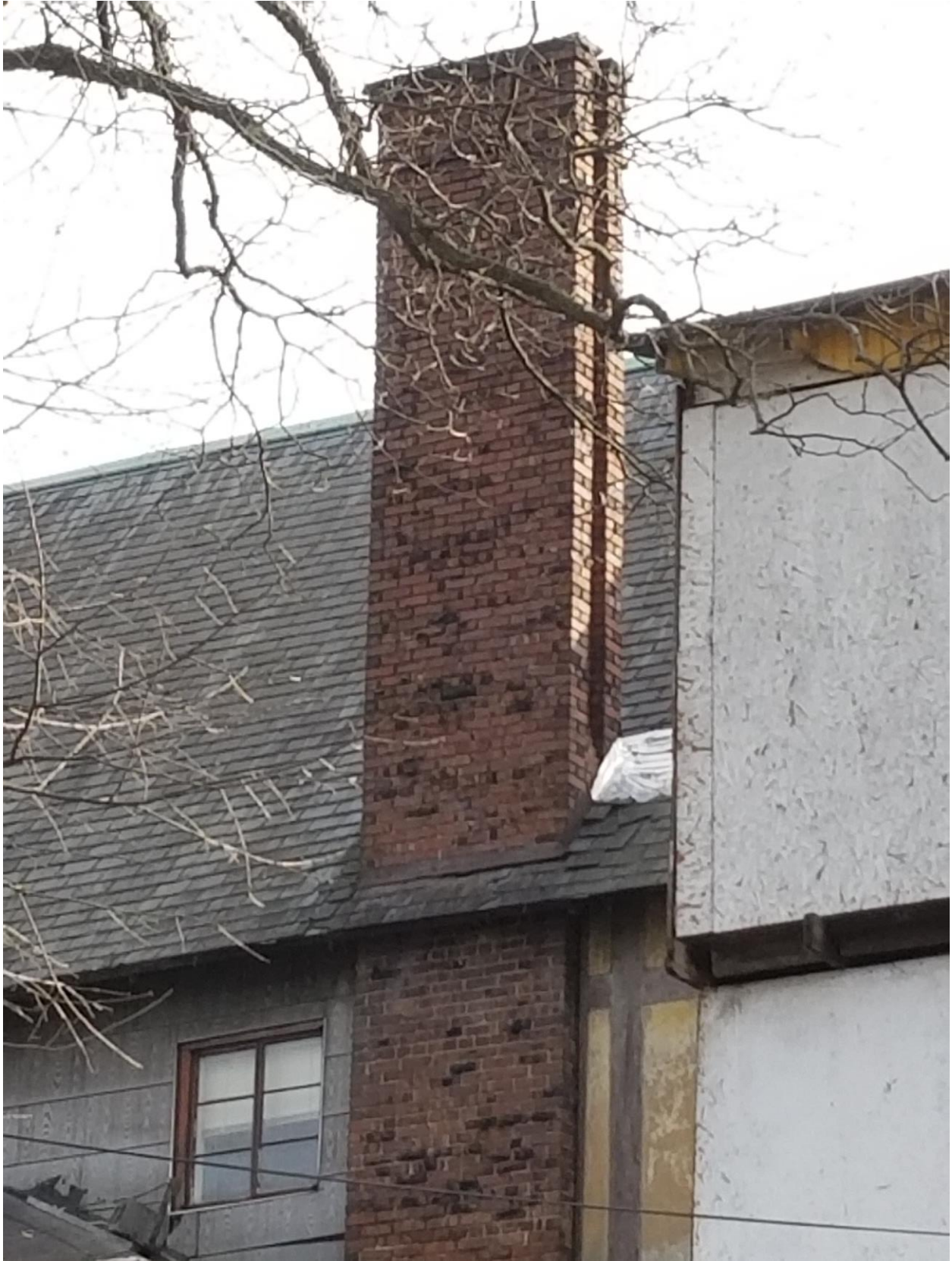
#23 – Upper portion of rear (north) façade and chimney detail, looking southeast
