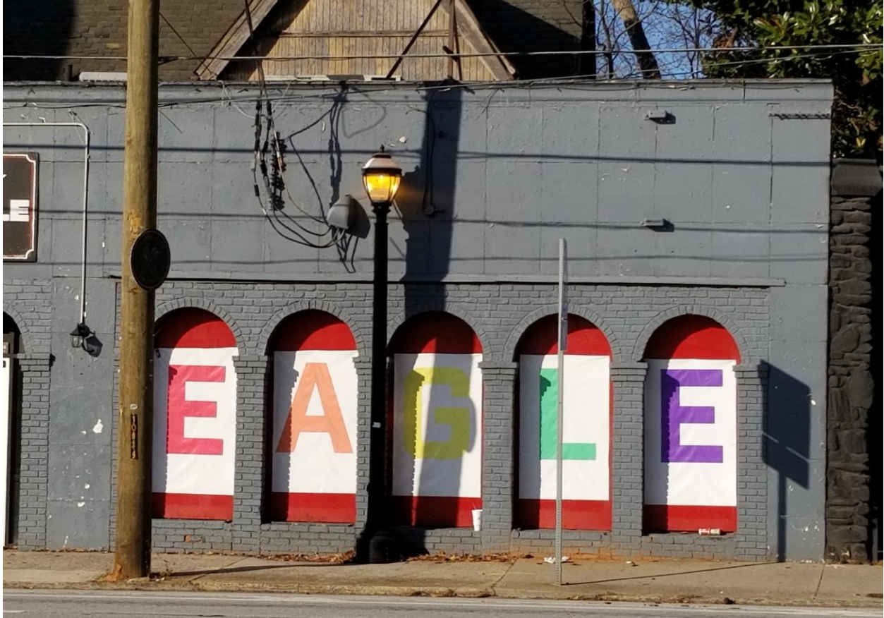
#5 – Lower east portion of front (south – Ponce de Leon Ave, NE) façade, looking north
